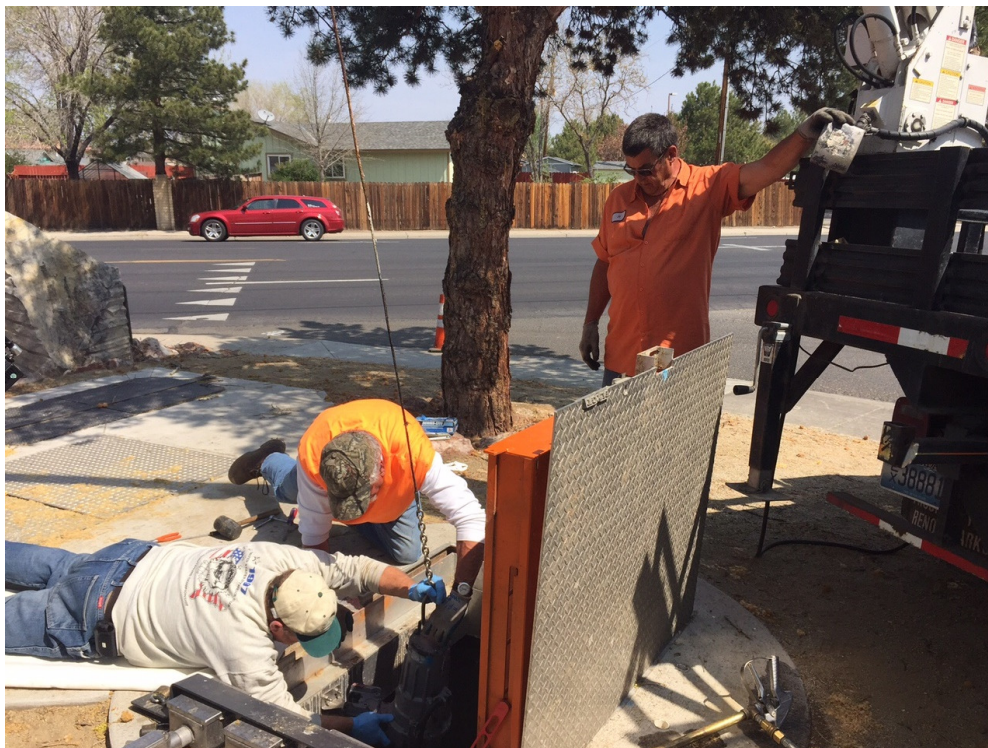
Sewer work on Prater Way
