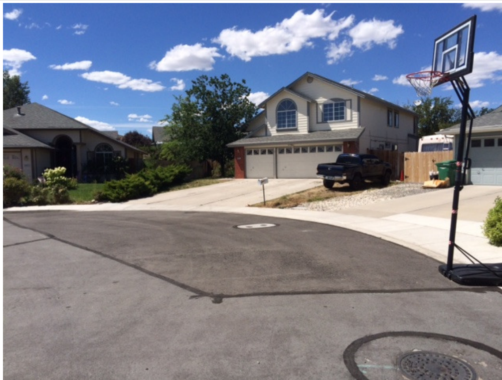
Street and sewer improvements on San Diego Court.
